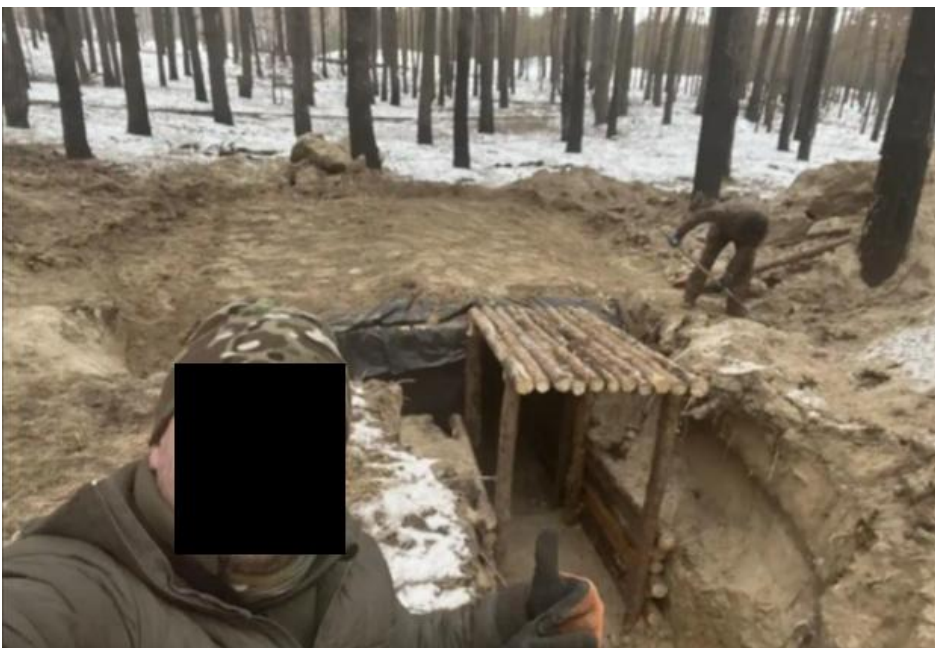
Figure 1. LT Volodymyr H. constructing a dugout
